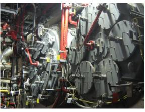
Custom engineered LE burners rated at 55 mmBtu/h HHV each are mounted on a field erected boiler wall. The burners are designed operate on 500°F combustion air and refinery fuel gas.
